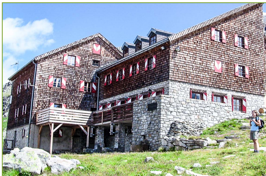
Fig. 89: All areas with permanent infrastructure were excluded from the wilderness zone.
