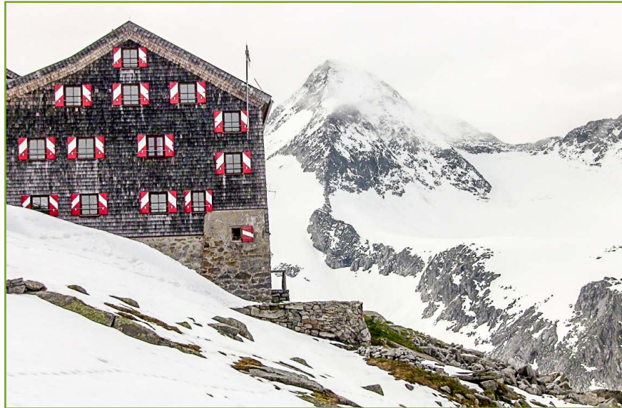
Fig. 90: Existing permanent structures provides also emergency service in low season (winter rooms).
